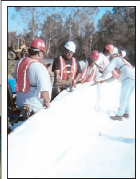
Sludge Lagoon Cap Reinforcement Installation Services
